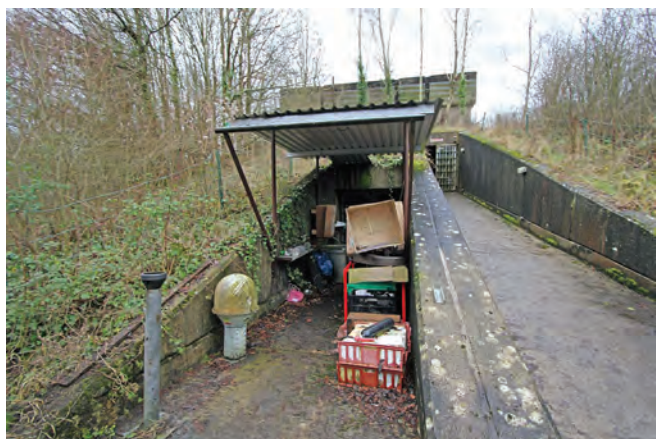
The main entrance blast door is up the ramp on the right. The ramp down on the left leads to another blast door. This is the machinery entrance at the rear of the generator room on the lower floor
